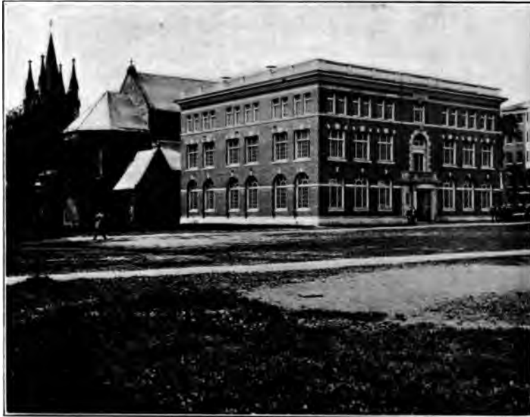
ST. STEPHEN'S CHURCH AND THE ENGINEERING BUILDING
